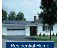
Residential Home Systems (2-8 kW)
