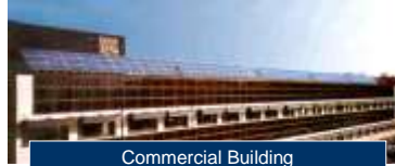
Commercial Building Systems (50 kW)
